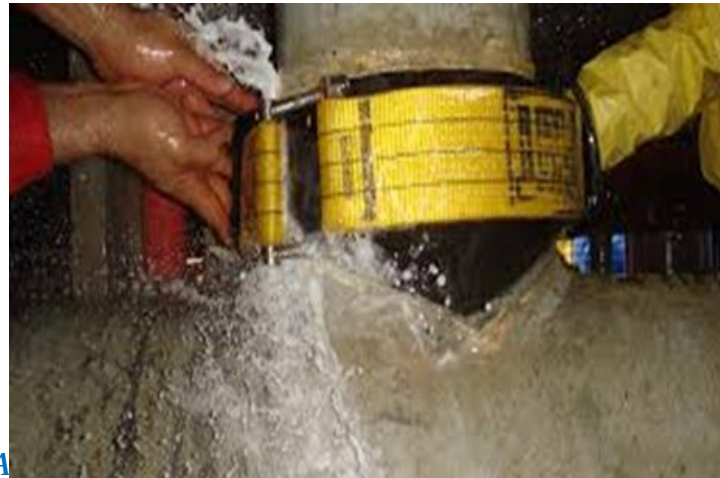
Online leak repairing
